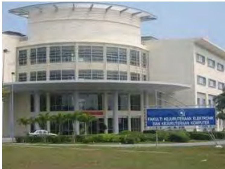
Fig. 2: KUTKM's new Campus
