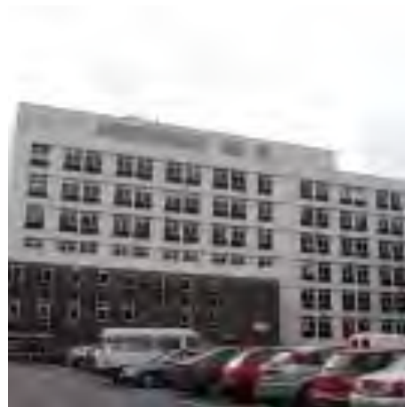
Fig. 5: Watts Building, Moulsecoomb
