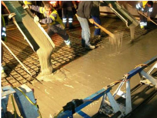
Figure 2.11 Strengthening of an industrial floor (Bruhwiler and Denarie, 2008)
