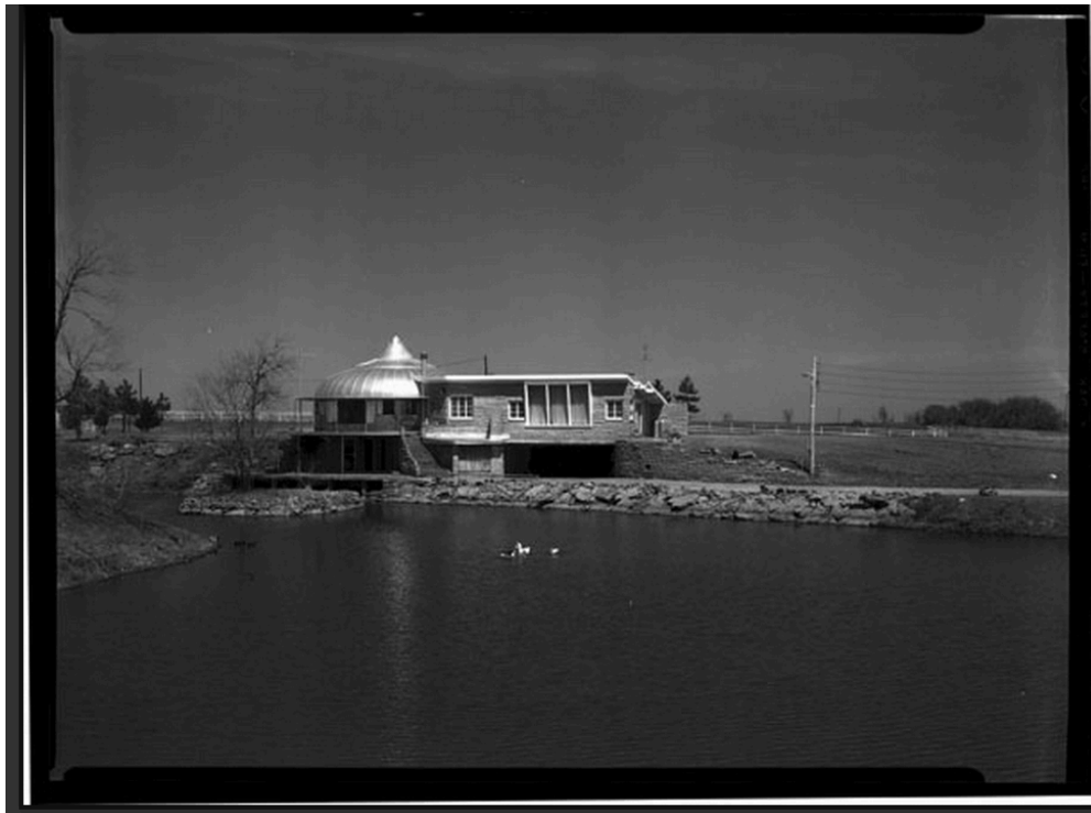
Figure 7: Graham family home incorporating modified "Wichita House," c. 1950 ( www.wichitaphotos.org )
