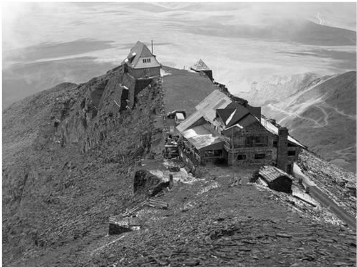
Figure 6.1 The Chacaltaya Research Station at 5260 m on Mt. Chacaltaya, Bolivia. Pictured is the building housing the laboratory (foreground) and the building where experimenters and participants resided during the project (background).
