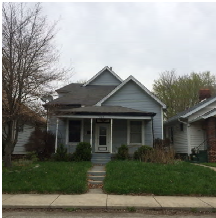
Figure 76: Example house for renovation around The Tube site (pre-renovation), Indianapolis, 2014. [Photograph].
