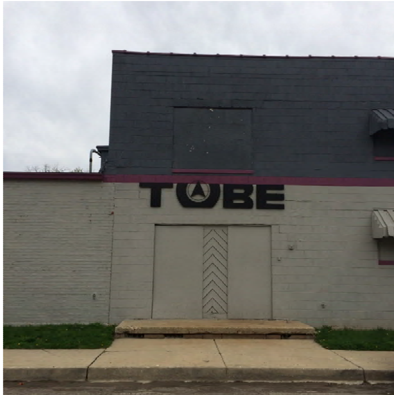
Figure 73: Exterior aspect of (the eponymous) The Tube warehouse (pre-renovation) from Nelson Street, Indianapolis, 2014. [Photograph].
