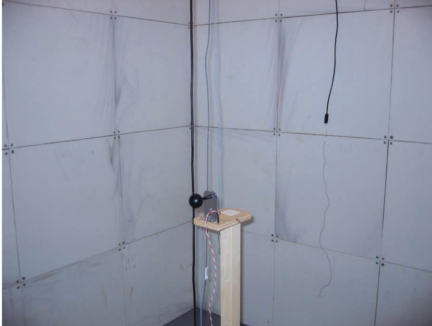
Figure 8.7 Internal view of Test Chamber containing phase change wall-lining and temperature monitoring equipment
