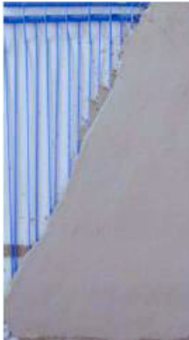
Figure 2.16 Maxit Clima PCM plaster applied over capillary cooling mats to produce an actively chilled ceiling (Fisch and Kühl, 2006)
