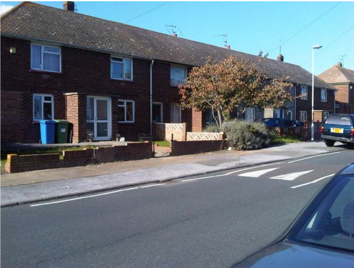
Figure 3.2: View of the un-retrofitted houses in Rushenden
