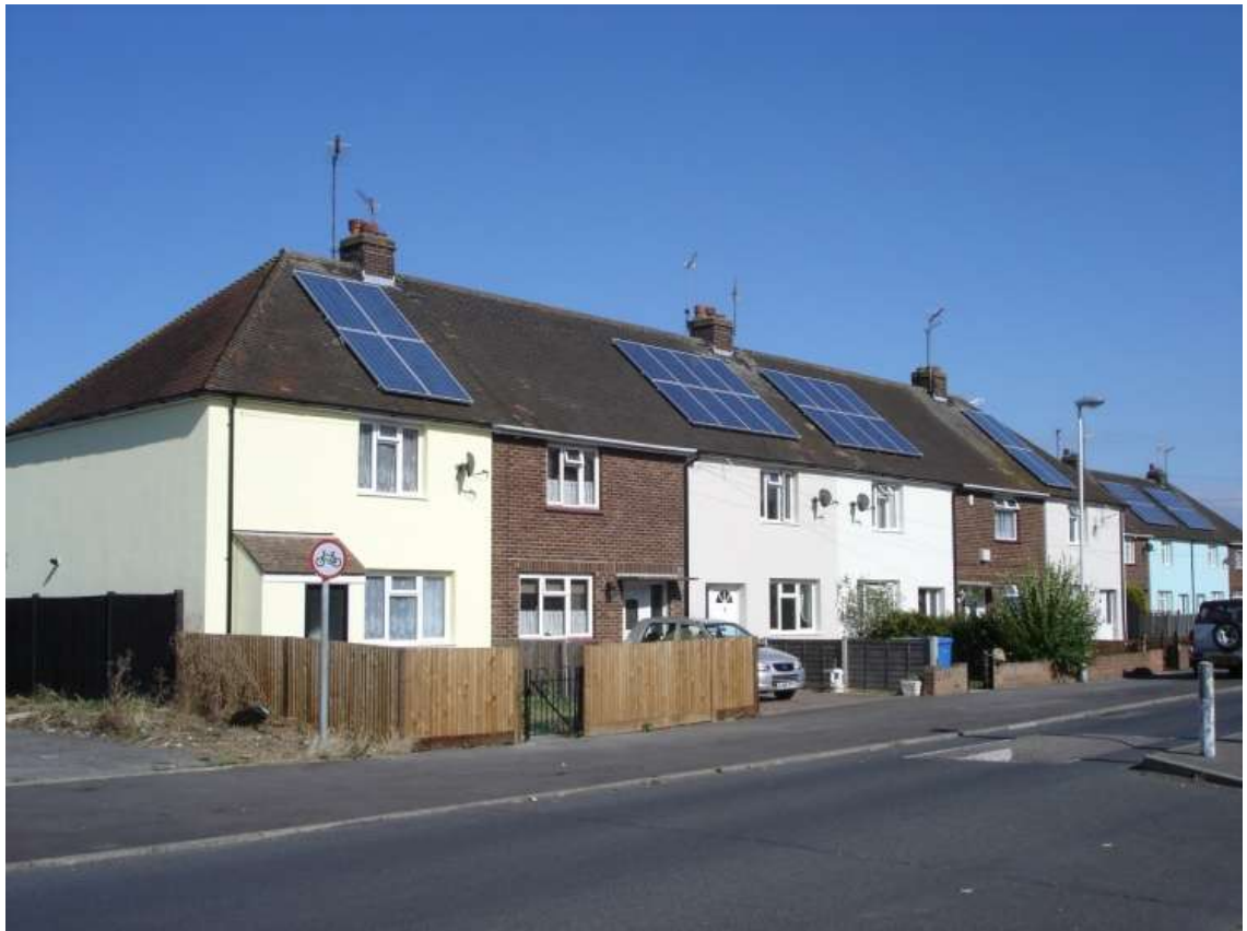
Figure 3.3: View of the retrofitted houses in Rushenden
