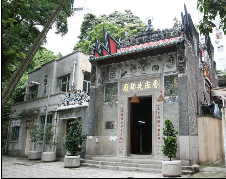
Figure 7. Lu Pan Temple, which has benefitted from the “Financial Assistance for Maintenance Scheme” for its repair work. (Source: www.heritage.gov.hk )
