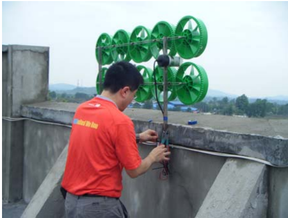
Figure 1-1 The micro wind turbine was installed at a reconstructed school in Sichuan.
