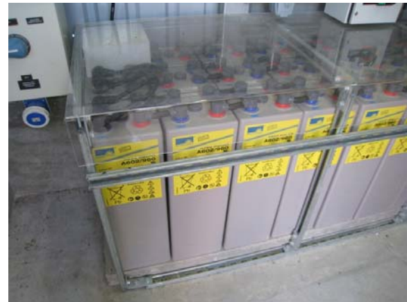
Figure 11-15 Batteries of the Town Island PV System
