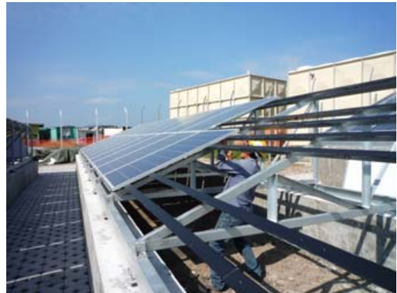
Figure 11-10 PV panel installation
