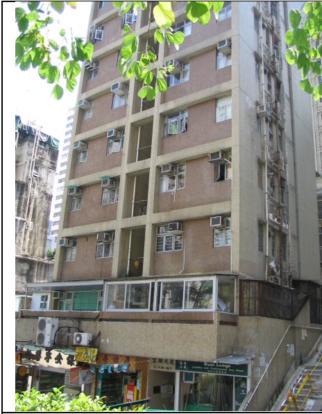
3a. Wide angle view of low-grade building
