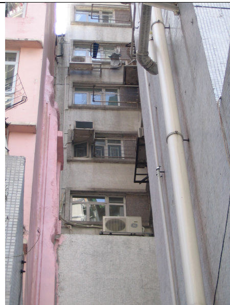
Close up view of medium-grade exterior
