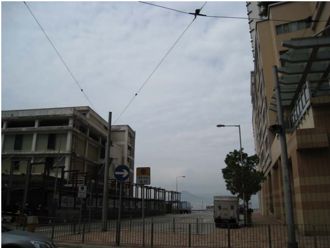
FIGURE 1: THE MERTON – No footbridge across Cadogan Street (Photo taken by author 13 th March 2008.)
