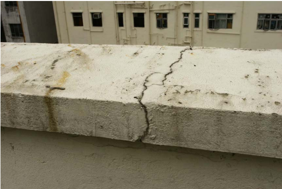
Figure 2.17 Concrete cracking
