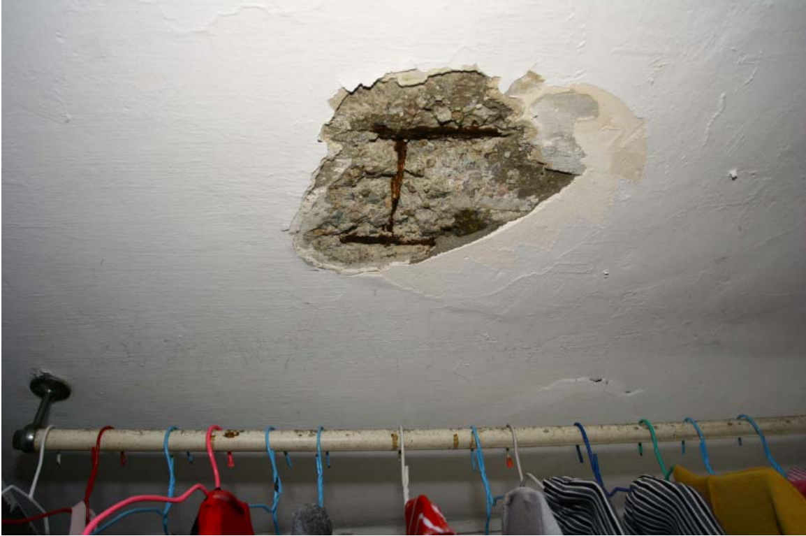
Figure 2.18 Concrete spalling
