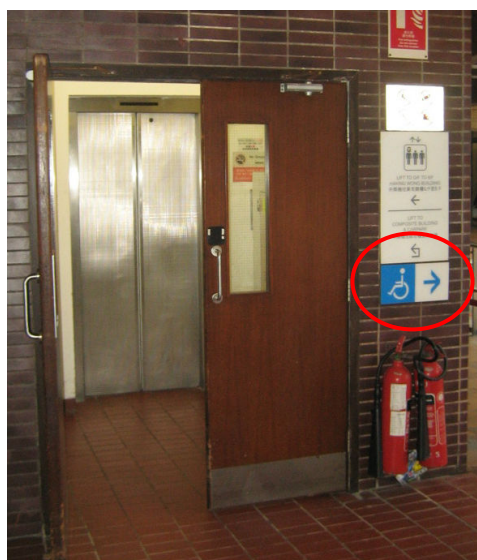
Pic. 39: Lift to G/F – 8/F of HW
