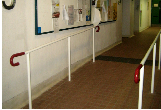
Pic. 58: Ramp with Two-side Handrails
