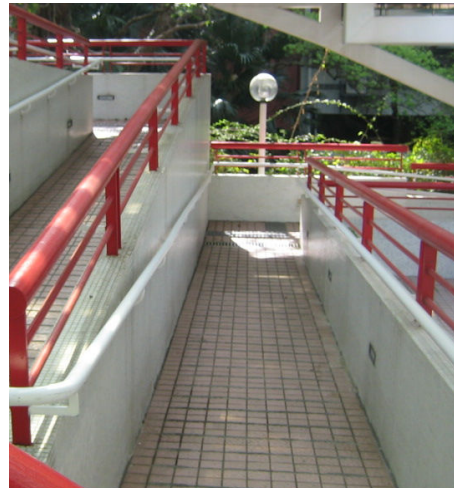
Pic. 66: Ramp to KK
