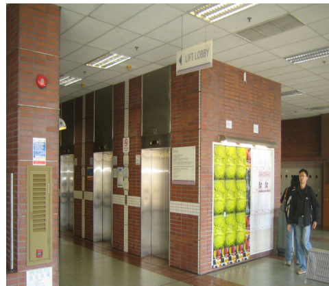
Pic. 4: Lifts to All Floors of CB
