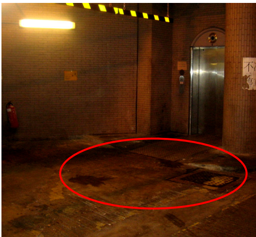
Pic. 56: Surrounding around Service Lift
