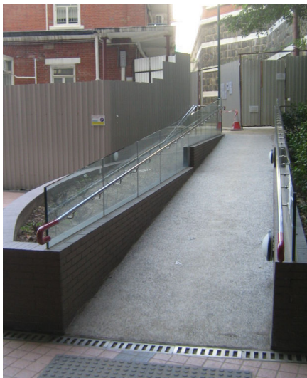
Pic. 20: Ramp outside EH
