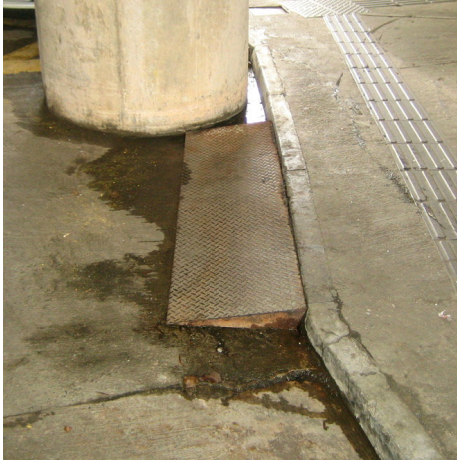
Pic. 73: Temporary Ramp from SWH to TC
