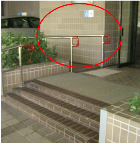
Pic. 69: Ramp at Entrance of KK
