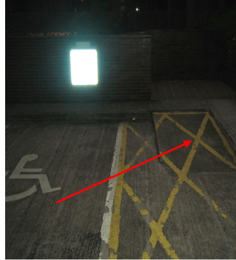
Pic. 89: Car-parking Space Designated for Wheelchair-bound Persons to RR/RM
