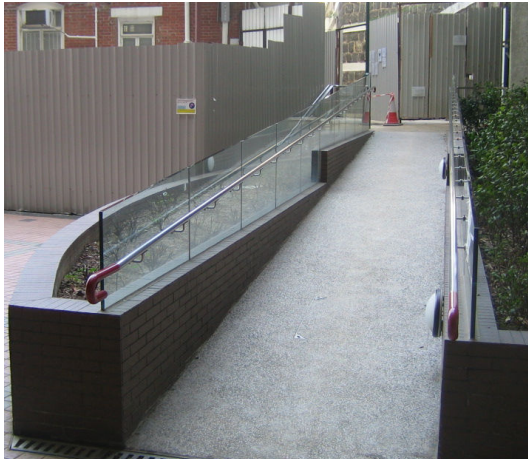
Pic. 61: Ramp with Two-side Handrails Leading towards EH
