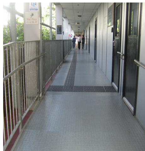
Pic. 10: Corridor on 5/F of HW to HC
