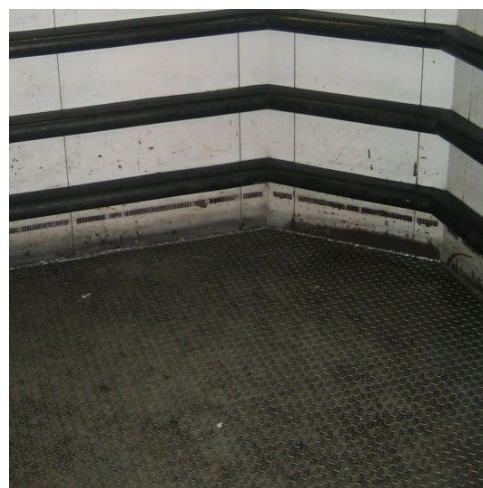
Pic. 57: Condition inside Service Lift
