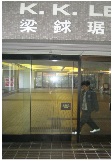
Pic. 67: Automatic Door at KK
