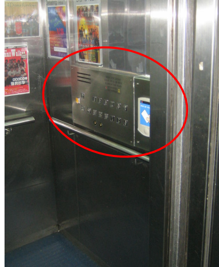
Pic. 34: Lift with Lowered Control Panel
