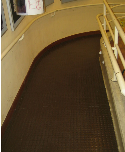
Pic. 33: Ramp with Two-side Handrails
