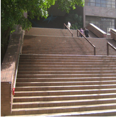
Pic. 29: Staircase at the West Gate
