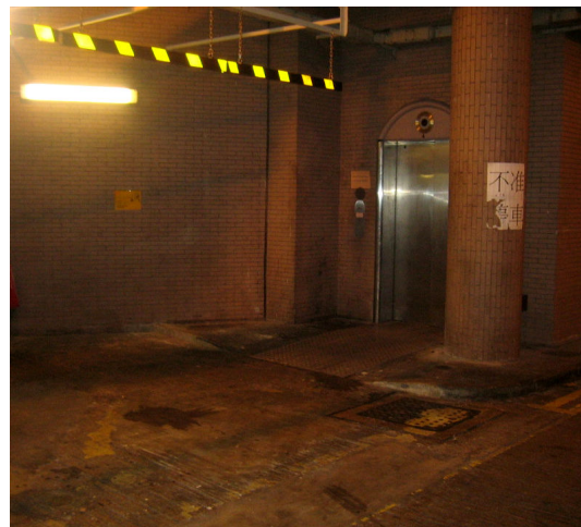
Pic. 18: Service Lift of Meng Wah Complex
