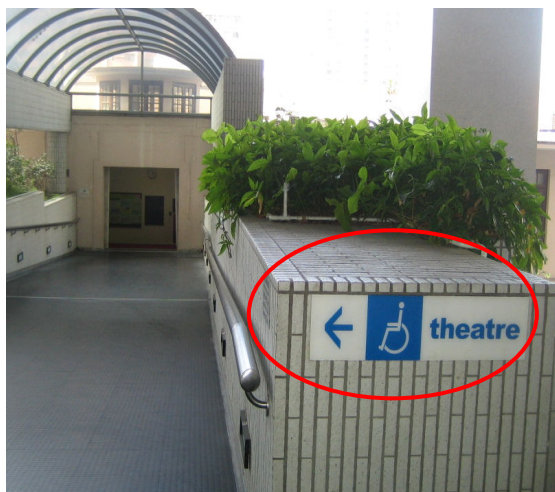
Pic. 82: Bridge from Library Extension to MB
