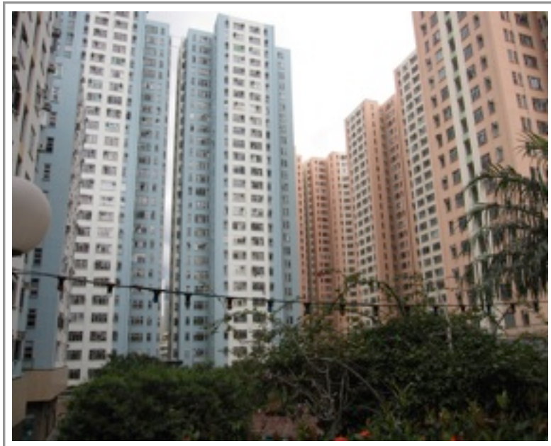
Block U and K in the northern side
