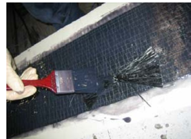
(b) Splying and epoxying of fan-out fibres onto fibre sheet
