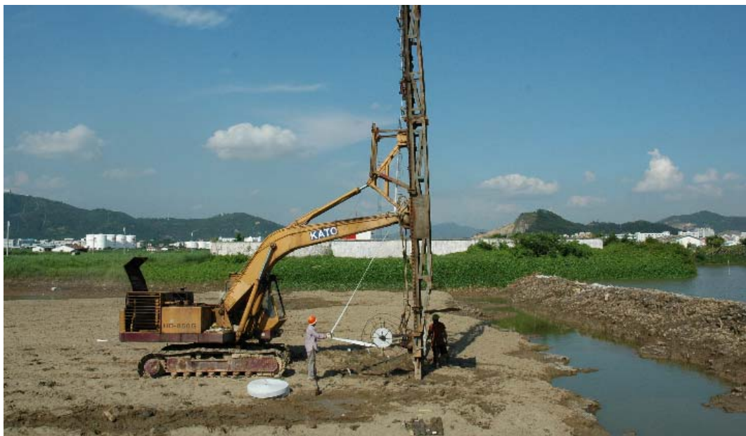
Fig. 2 Installation of Wick Drains
