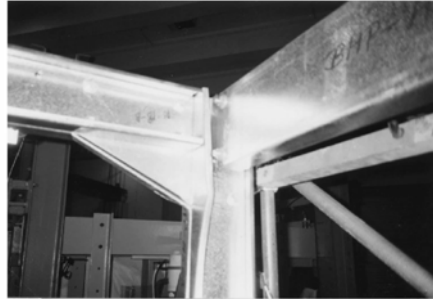
Figure 4. Typical web buckling induced failure [Ref. 14]
