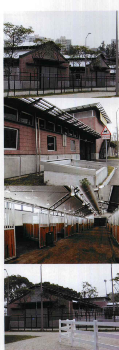
马厩外观与内部 1 External view and interior of stables, 1
