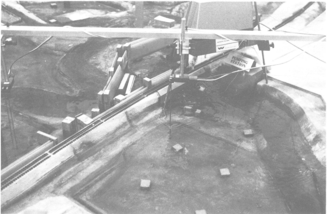
Fig. 4 Submergence of the soffit of the railroad bridge at the Indus
