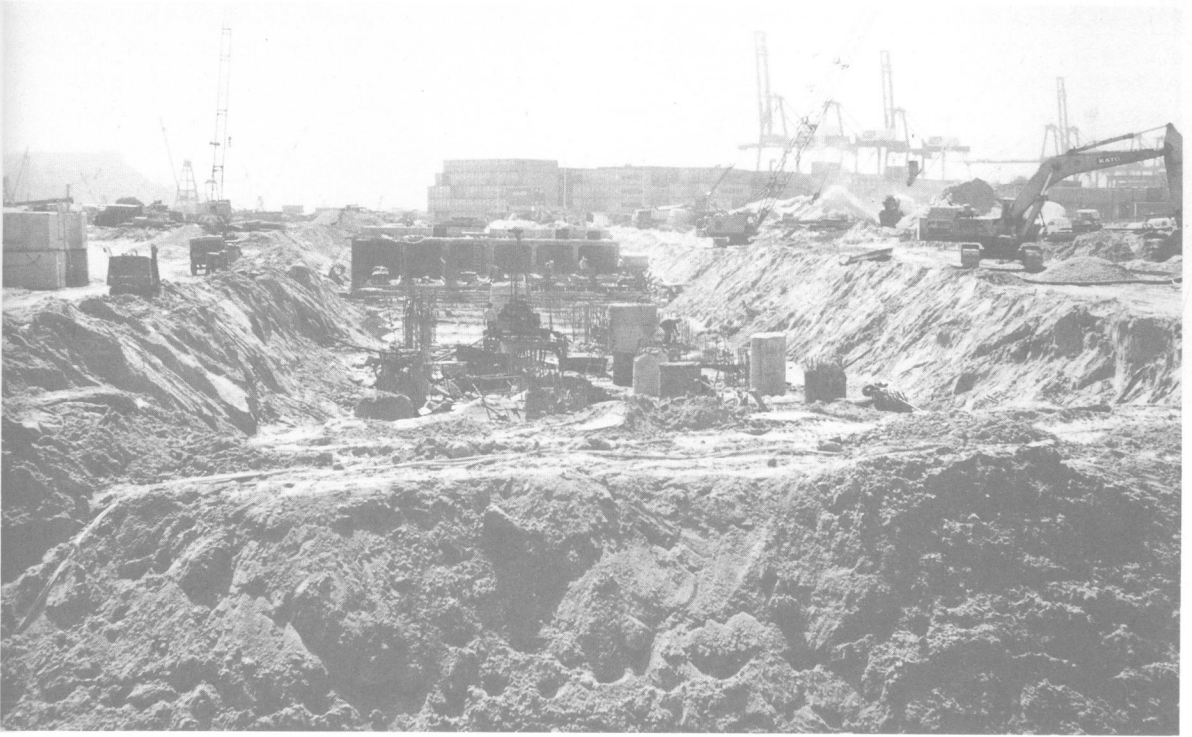
Plate 2 Formation of a multiple-cell box culvert on the West Kowloon Reclamation.
