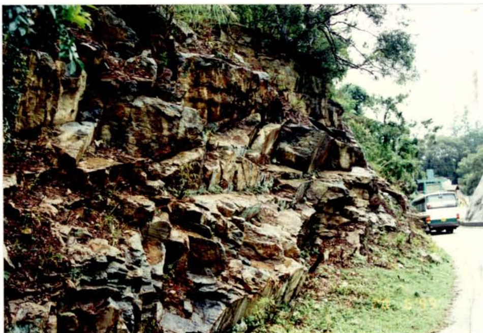
Plate 5.1. Jointed volcanic rock exposed after roadcutting at Keung Shan Road
