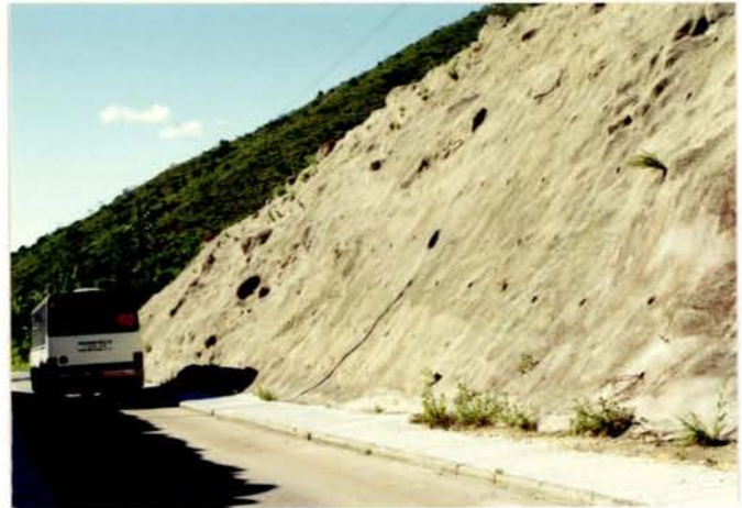
Plate 9.3. Roadcuts along Tung Chung Road
