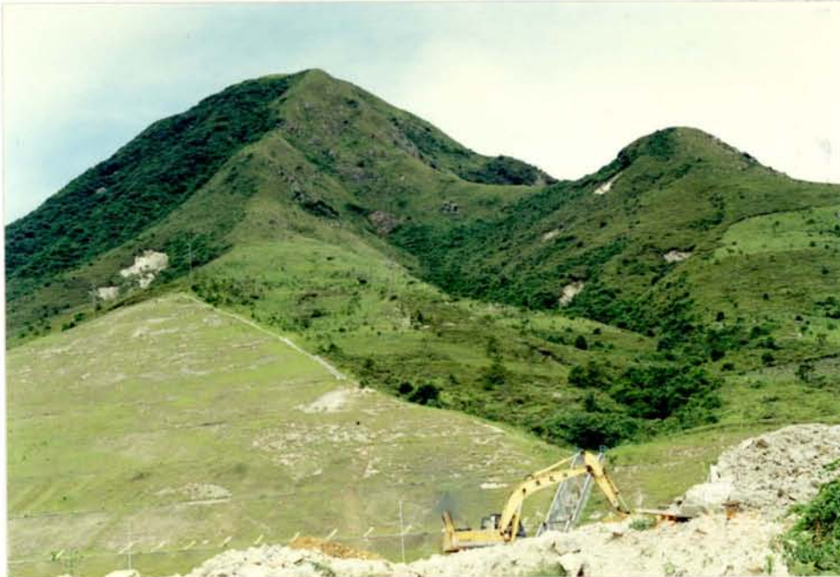
Plate 9.5. Landslides on natural hillslopes above a roadcut, Tung Chung
