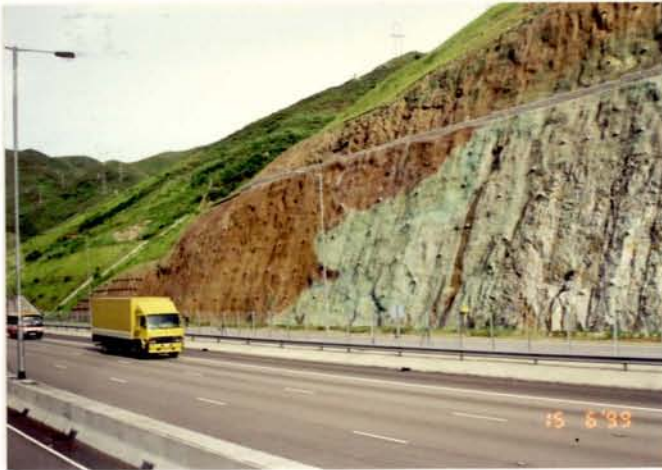
Plate 9.2. Steep roadcuts along the North Lantau Expressway
