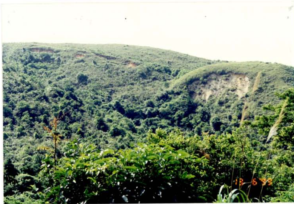
Plate 7.7. Landslide scar under revegetation on a steep slope beside Tung Chung Road
