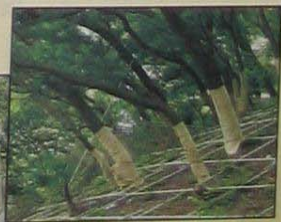
在工程中保護斜坡上的樹木 Protect trees on slopes during construction
