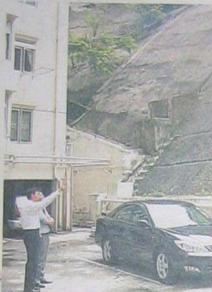
▲ 提供維修意見 Advice on Slope Maintenance Works
