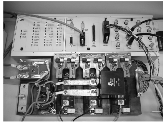
Figure 13. The power converter and dSPACE connector/led panel.
