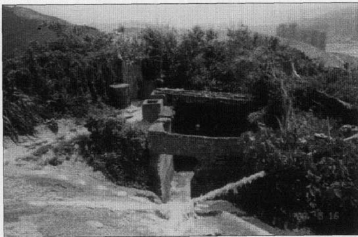
Plate 3 Improvised steel water tanks, water pipes and a shed found in one of the bunkers inside the Devil’s Peak Redoubt
