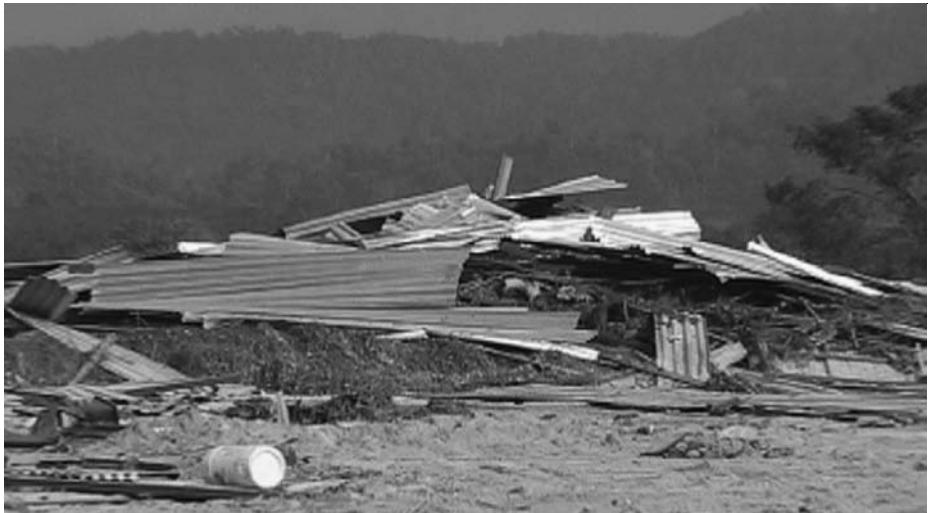
Plate 2. Floating debris injured or buried victims. Collapsed sheet-metal walls and roofing were lethal
