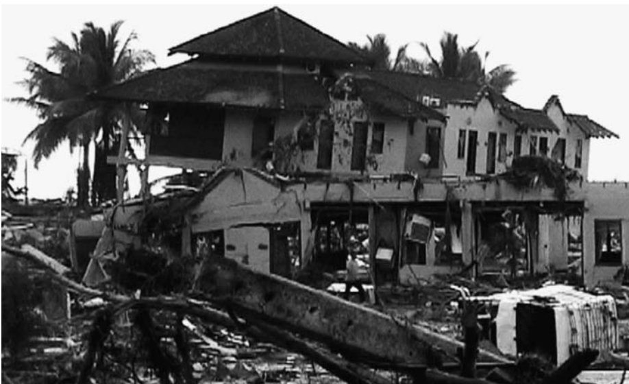
Plate 3. Beachside hotels took the full impact of the wave. This Khao Lak hotel was lifted off its foundations
