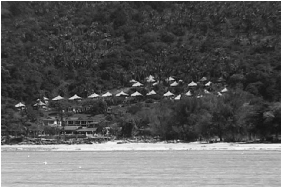
Plate 4. A Phi Phi resort that survived was a few meters above sea level
