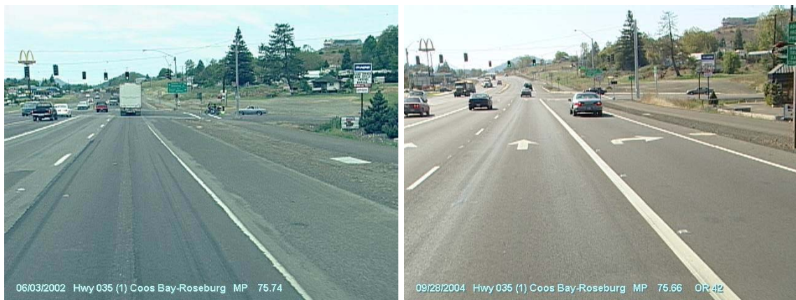
Figure 5.4: Conditions in 2002 (before) and in 2004 (after) showing the addition of the right-turn lane at “Kelly’s Corner” MP 75.72. OR-99 improvements not shown.
