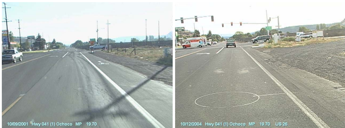
Figure 5.27: Conditions in 2001 (before) and in 2004 (after) showing the traffic signal installation at OR 126 and Combs Flat (MP 19.75)
