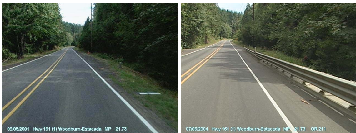
Figure 5.29: Conditions in 2001 (before) and in 2004 (after) showing the added guardrail/upgraded culvert at Milk Creek (MP 21.73)
