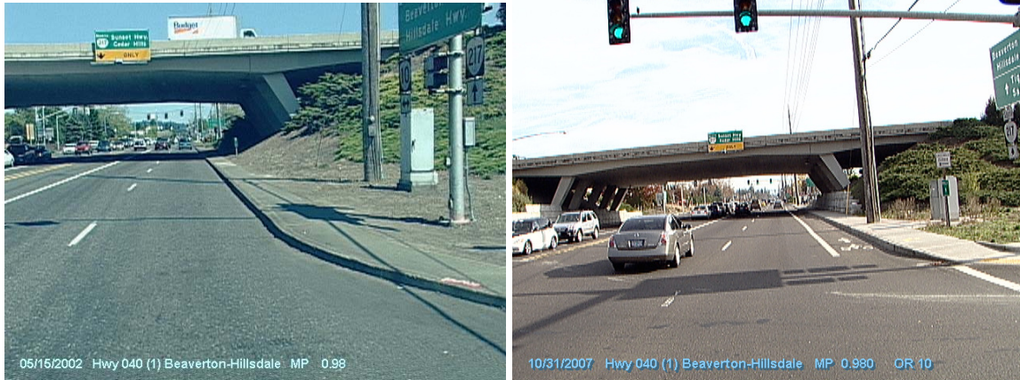
Figure 5.42: Conditions in 2002 (before) and in 2007 (after) showing construction at MP 0.98. Dual-left turn lanes at next connection not shown.
