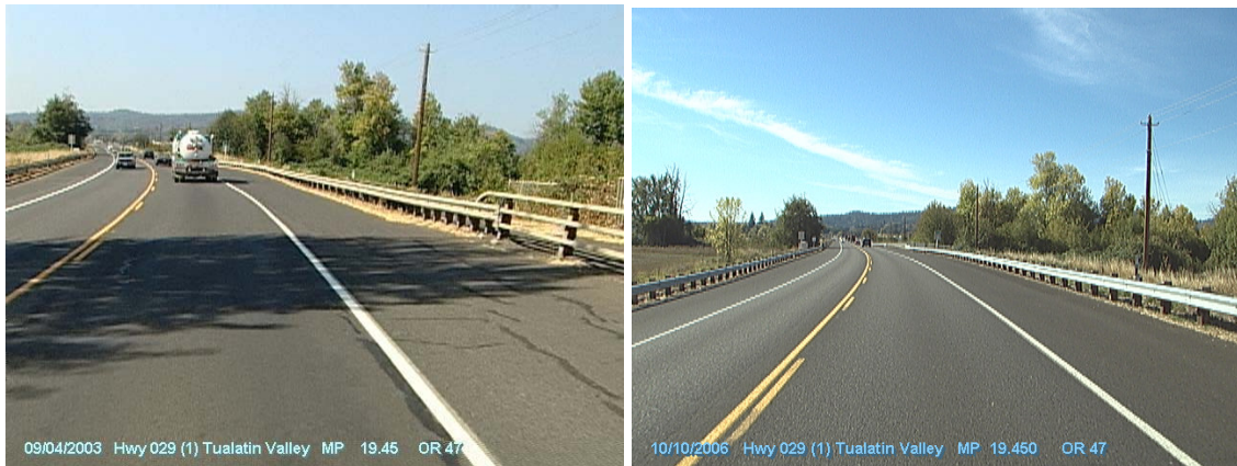
Figure 5.15: Conditions in 2003 (before) and in 2006 (after) showing the upgraded guardrail at MP 19.45
