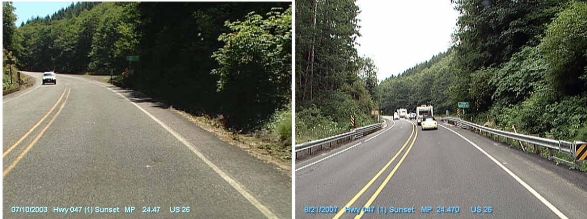
Figure 5.40: Conditions in 2003 (before) and in 2007 (after) showing the upgraded guardrail at Bridge No. 02166 at MP 24.47
