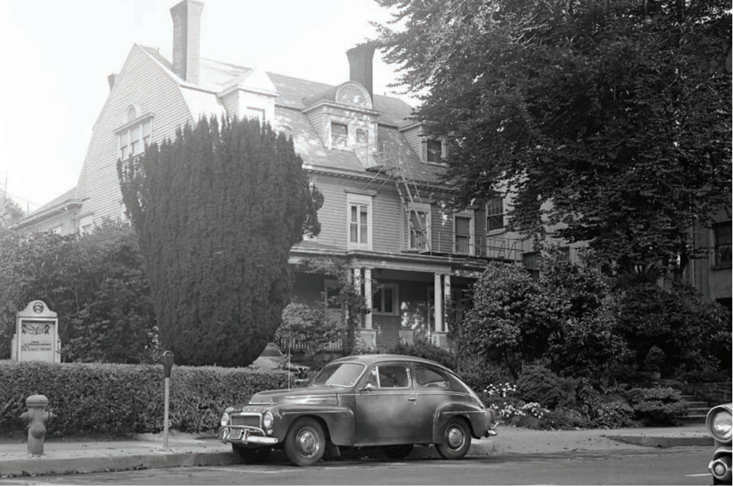
ABOVE The Watson's family home with the Beech tree in the upper right, Park and Hall Streets. Houses for condemnation, September 16, 1965, University Archives, Portland State University Library.
