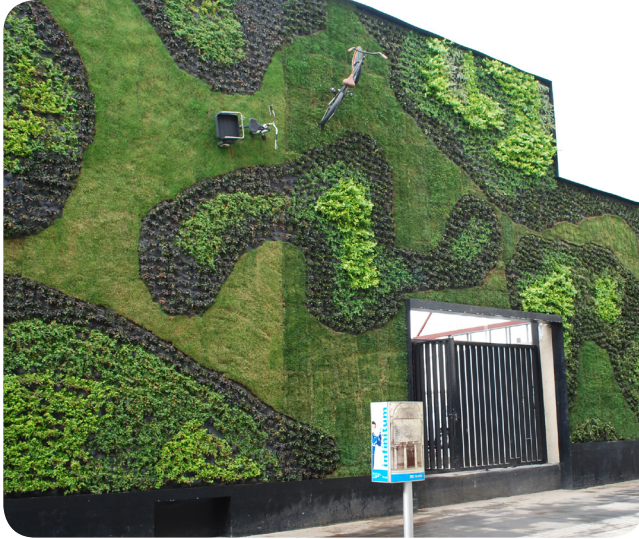
Image 15: Green wall in Mexico City, Mexico
