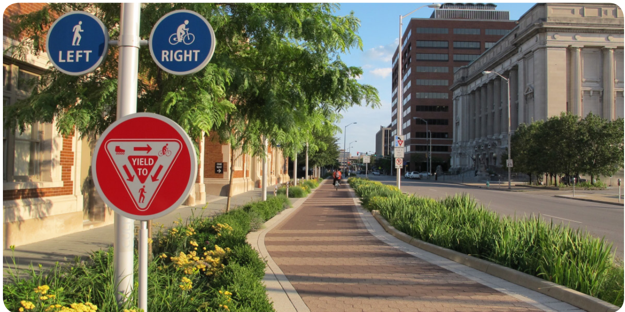
Image 2: The Indianapolis Cultural Trail features separated facilities and illustrates the prioritization of slower modes
