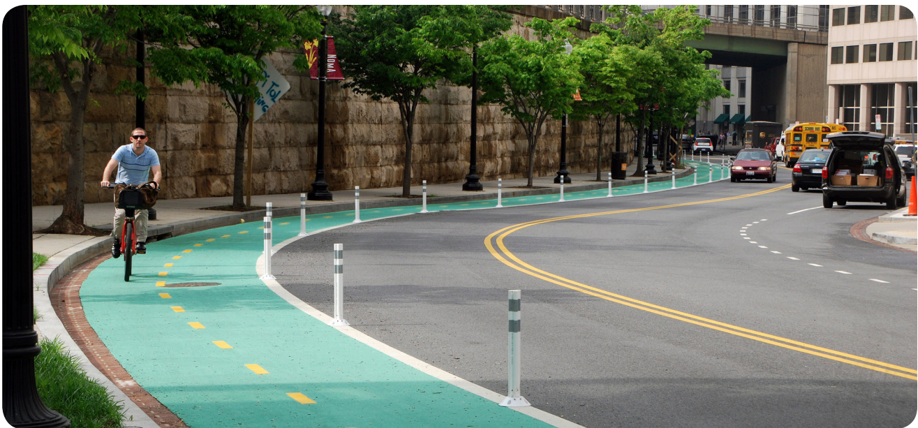
Image 29: Flexiposts create vertical physical separation between bicycles and cars in Washington DC.
