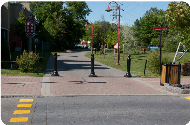
Image 26: Bollards create a symbolic barrier in Quebec, Canada
