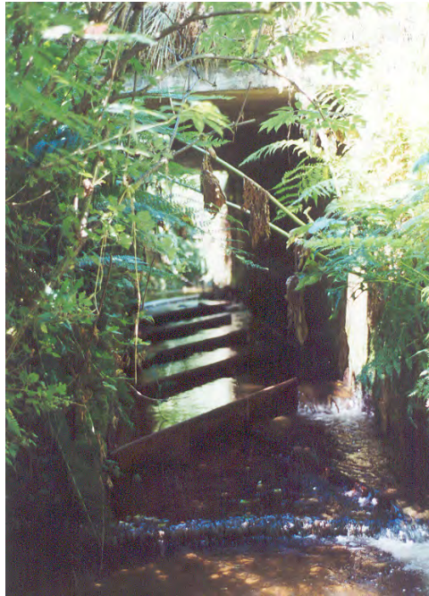
Figure 2.1: Example of Baffles in a Box Culvert
