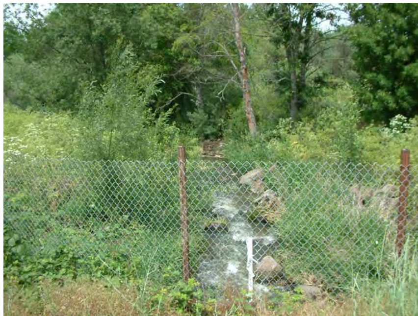
Figure 4.8: Site 06 – Roughened channel at Griffin Creek
