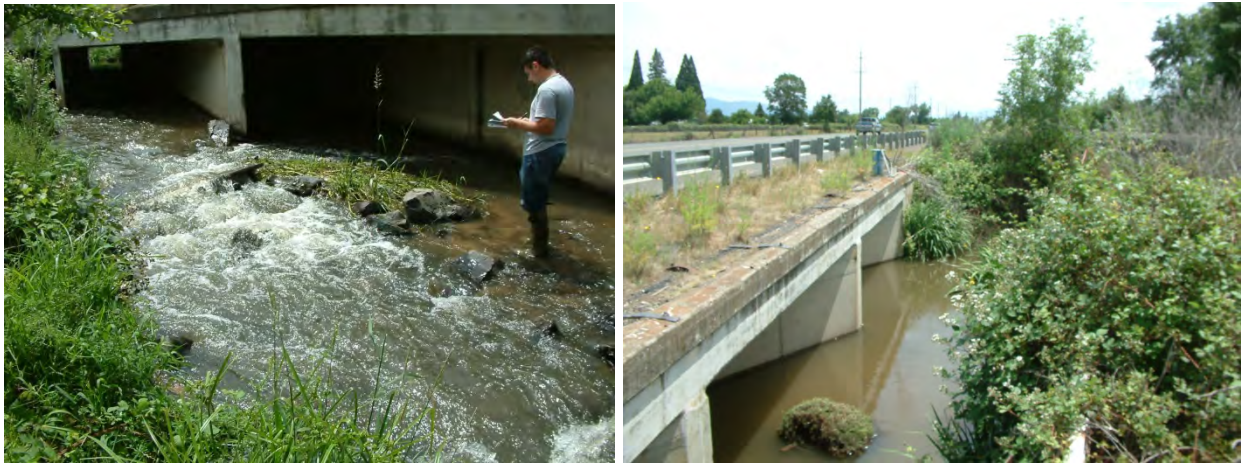
Figure 4.9: Site 07 - Jackson Creek (1) downstream and upstream
