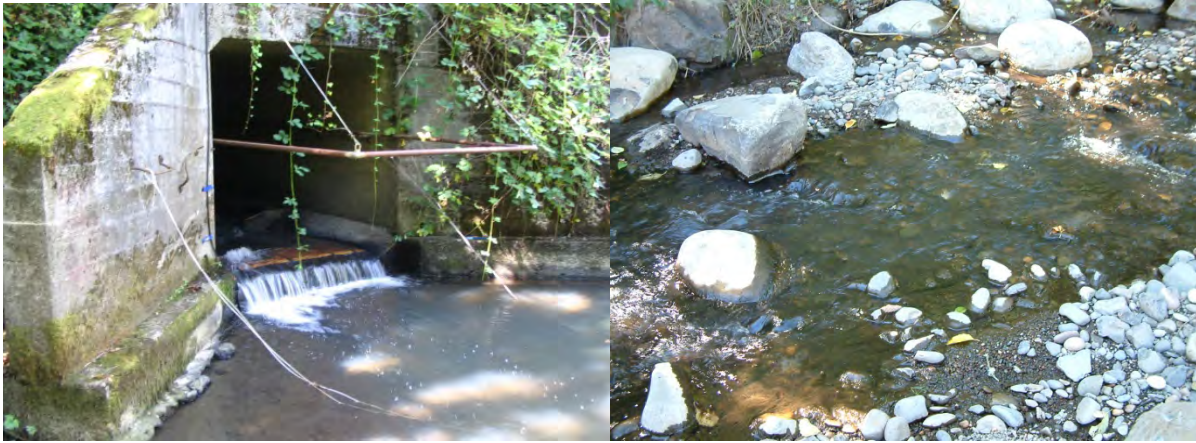
Figure 4.19: Site 17 - Tryon Creek outlet and downstream
