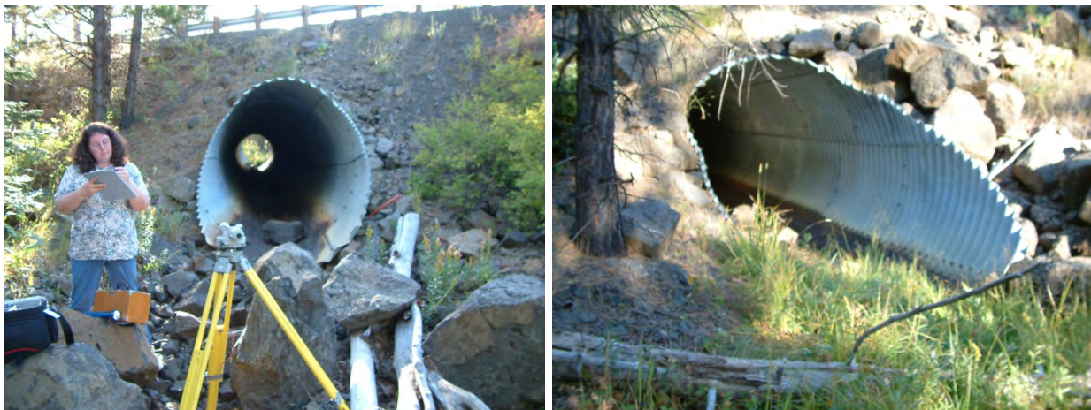
Figure 4.23: Site 21 - Porter Creek downstream and upstream
