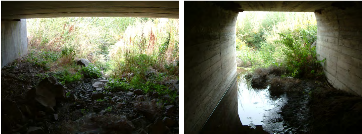
Figure 4.24: Site 22 - Stewart Creek – Culverts under new and old highways
