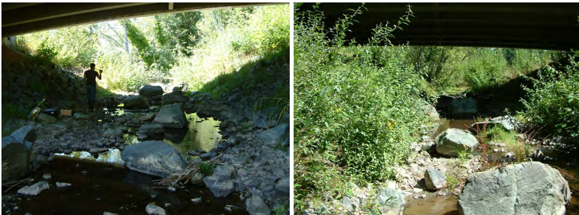
Figure 4.16: Site 14 - Bethel Creek under structure and downstream
