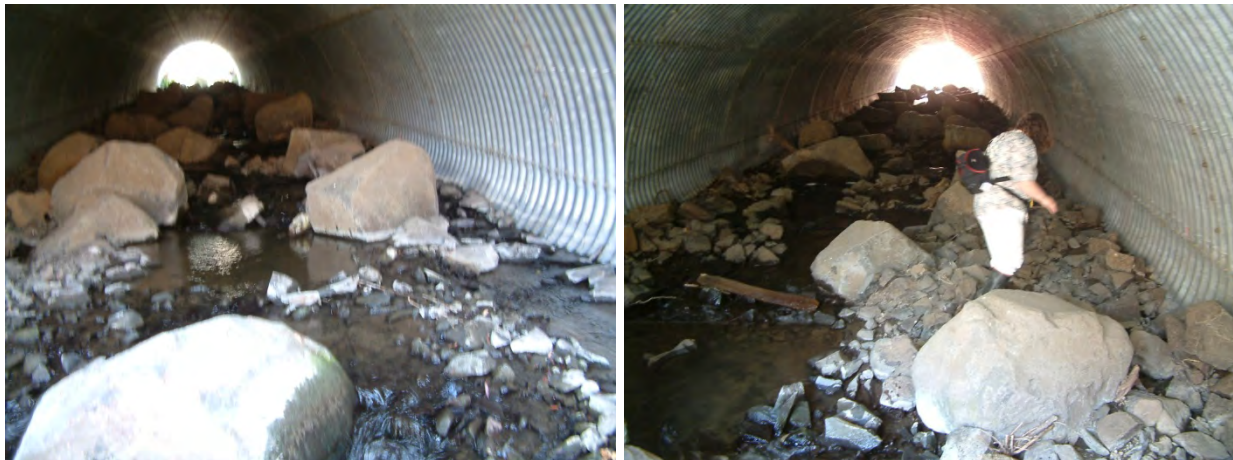
Figure 4.21: Site 19 - Three Mile Creek structure looking downstream and upstream
