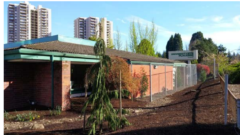
The retail building on the "Wyse" parcel
