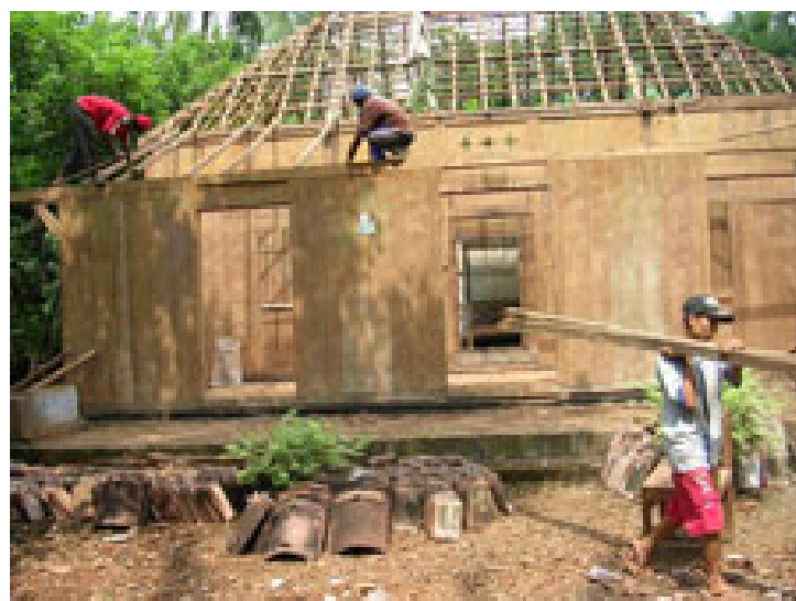
House deconstruction site
