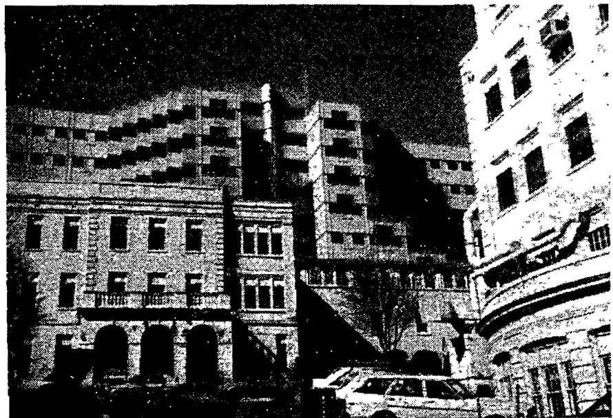
New Veterans Administration Hospital in background. Older Buildings to be removed for a Parking Structure.
