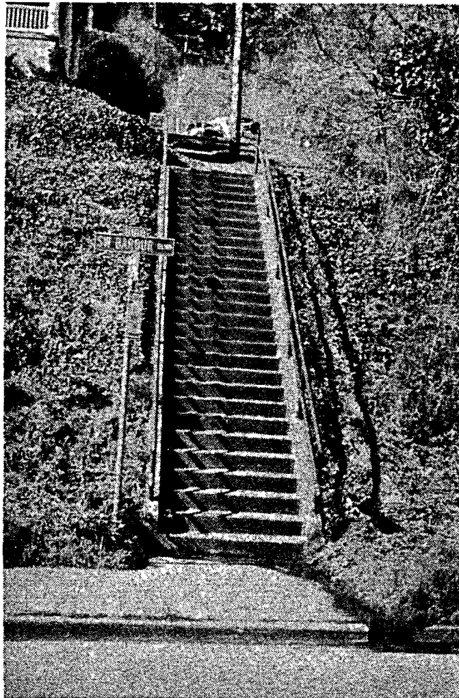
Stairs dead end at bottom of Lowell St. at Barbur Blvd.
