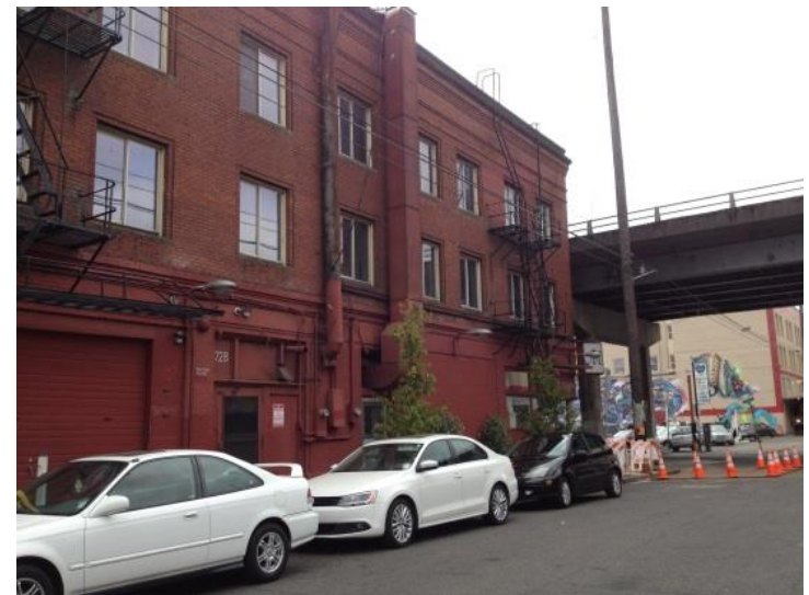
Figure 16 Royal Hotel looking south
