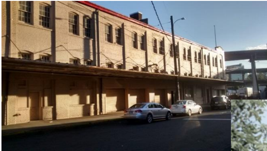
Figure 25 View of Alder Building looking west on Alder
