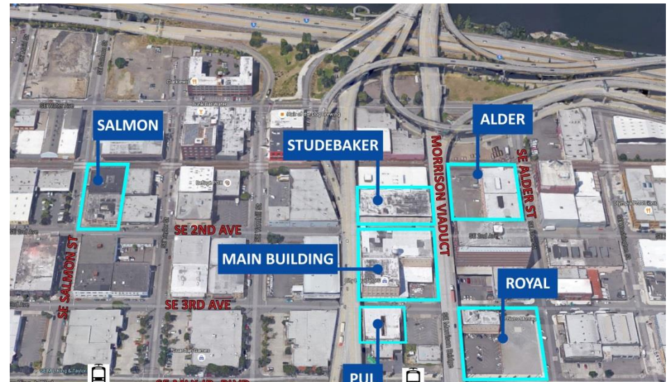
Figure 3 Aerial Photo of Pelett Properties
