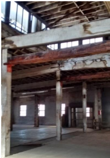
Figure 12 Alder Building Clerestory Windows and Large Wood Beams
