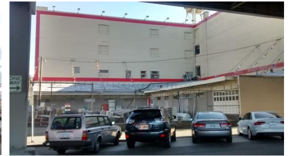
Figure 6 Main Store Storage at corner of SE 3 rd and Morrison
