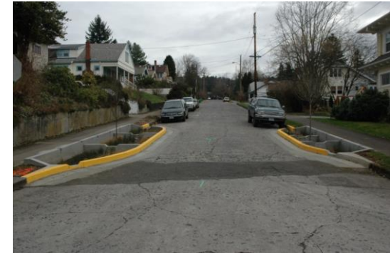
East Portland bioswales
