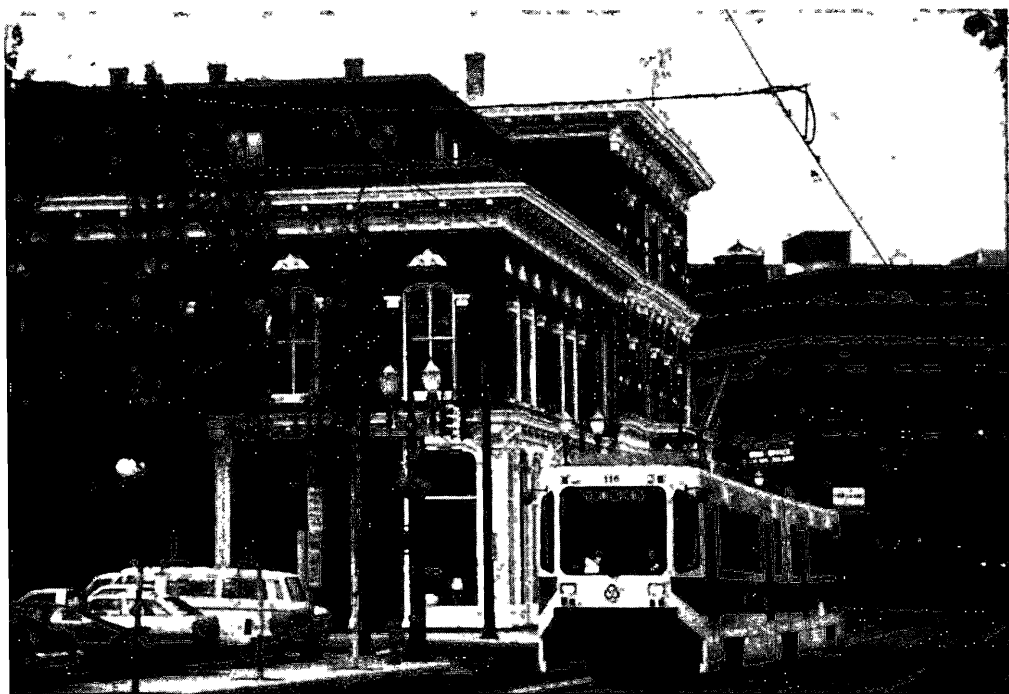
Figure 4.6: New Market Theatre Building with MAX light rail train on S. W. 1st Avenue in the Skidmore-Old Town Historic District. The New Market Theatre (high white facade) was originally built as a produce market with a grand theater on the second floor. For much of the 20th century a parking garage, it was recently restored as a shopping arcade with offices on the upper floors (Photo: John V. A. F. Neal).
