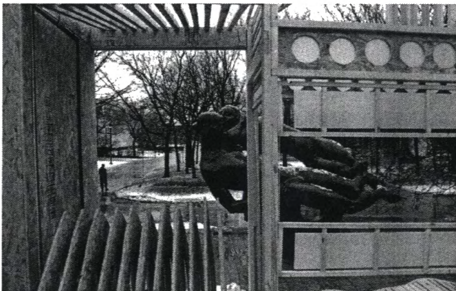
Fig. 3. A detail showing the connection between three cells of the entire structure.
