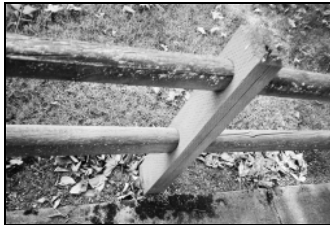
Figure 91: On both sides of the fence.
