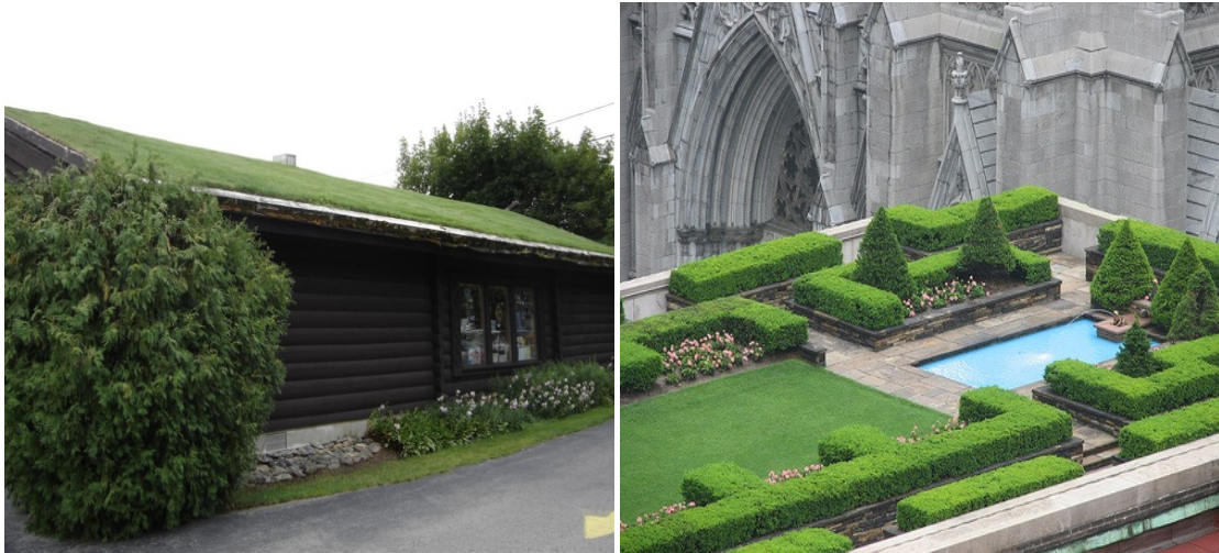
Figure 1 Intensive roofs (right) and extensive roofs (left)
