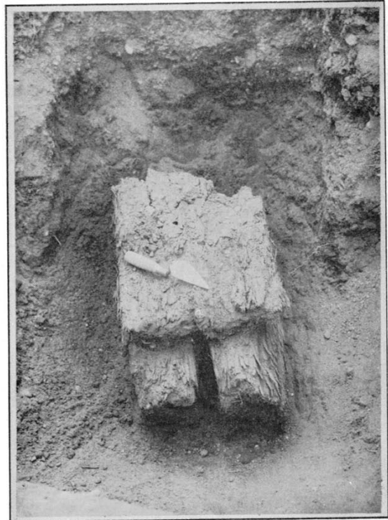
B. Block footing found in northeast corner of Chief Factor's house.
