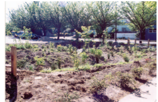
The St. Philip Neri bioswale manages all stormwater runoff from adjacent surface parking lot
