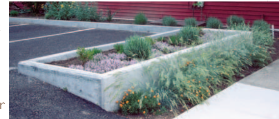
Stormwater planters and porous pavement at Full Health Spectrum, located at SE 32nd and Division
