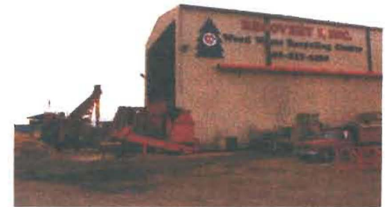
Recovery One in Tacoma, WA
