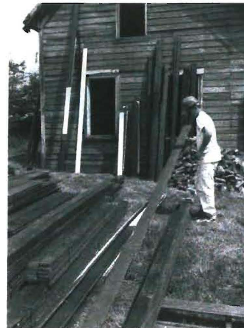
Sorting used lumber after house deconstruction
