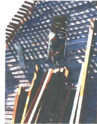
Deconstruction in progress
