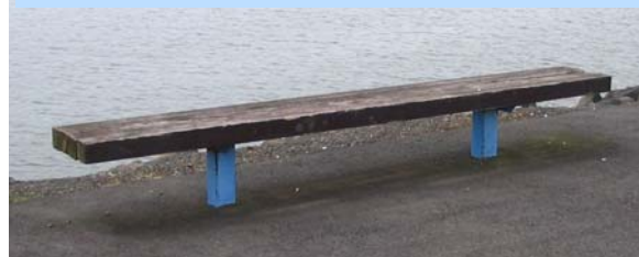
Although a few benches are located along the pathway, they are worn and look uncomfortable.
