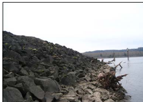
Rip rap along the North site
