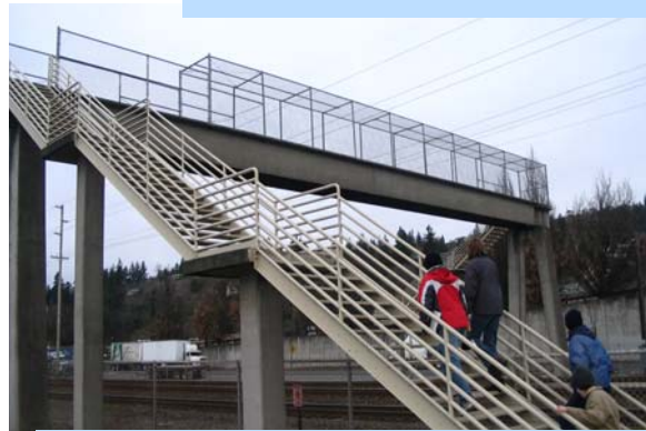
Pedestrian overpass has steep metal staircase and is covered with fencing.
