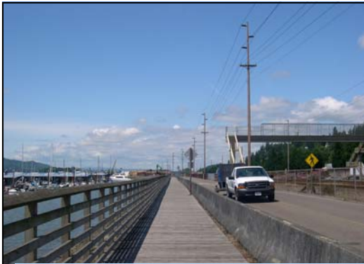
Existing boardwalk is separated from Hendrickson Drive with unattractive jersey barriers. A high wooden railing compliments boardwalk but inhibits views.
