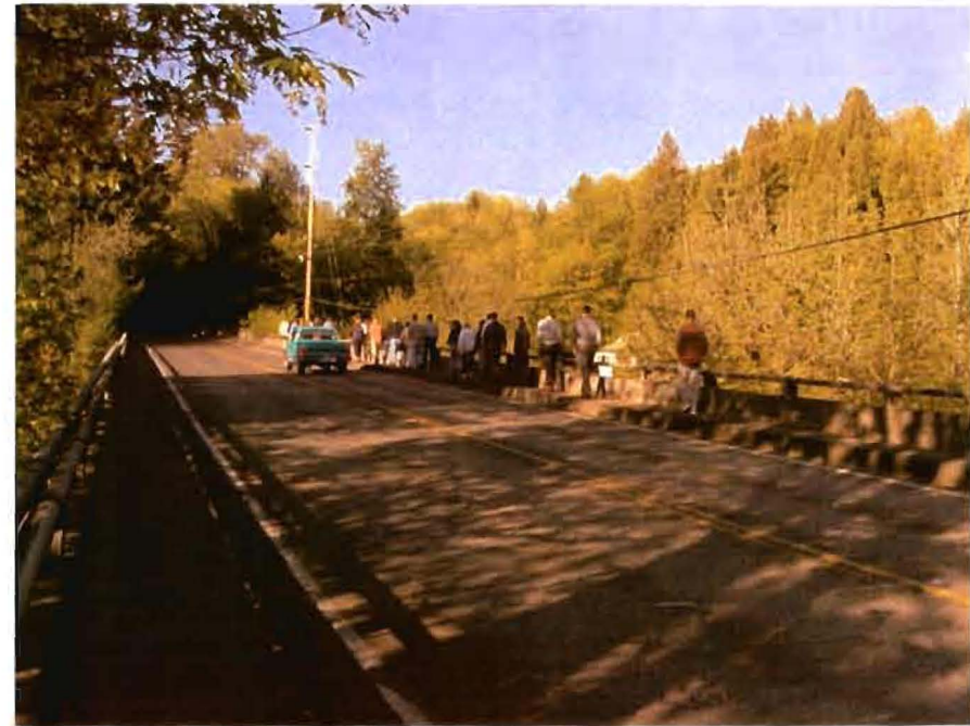
Bridge Over Tualatin River, Stafford Road
