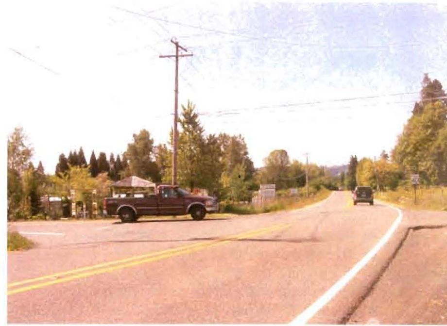
Intersection of Rosemont Rd. and Stafford Rd.
