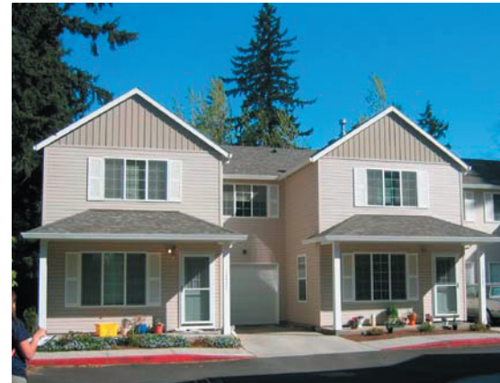
Boise Street Condos provide a clear transition between the private and public environment with porches, front yards and sidewalks.
