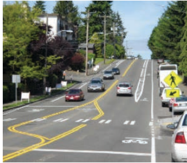
Figure 30. Before & After Buffered Bike Lane in Seattle
