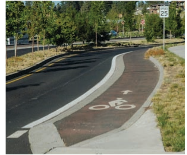
Figure 31. Raised Bike Lane in Bend, OR
