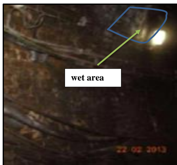
Figure 3-106 TL56 visual inspection wet area (LUL, 2011)
