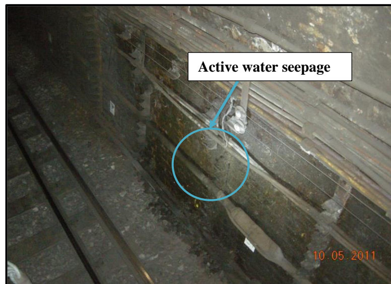
Figure 3-78 TL17- active water seepage at chainage 77, from the arch springer to track level- visual inspection 2013
