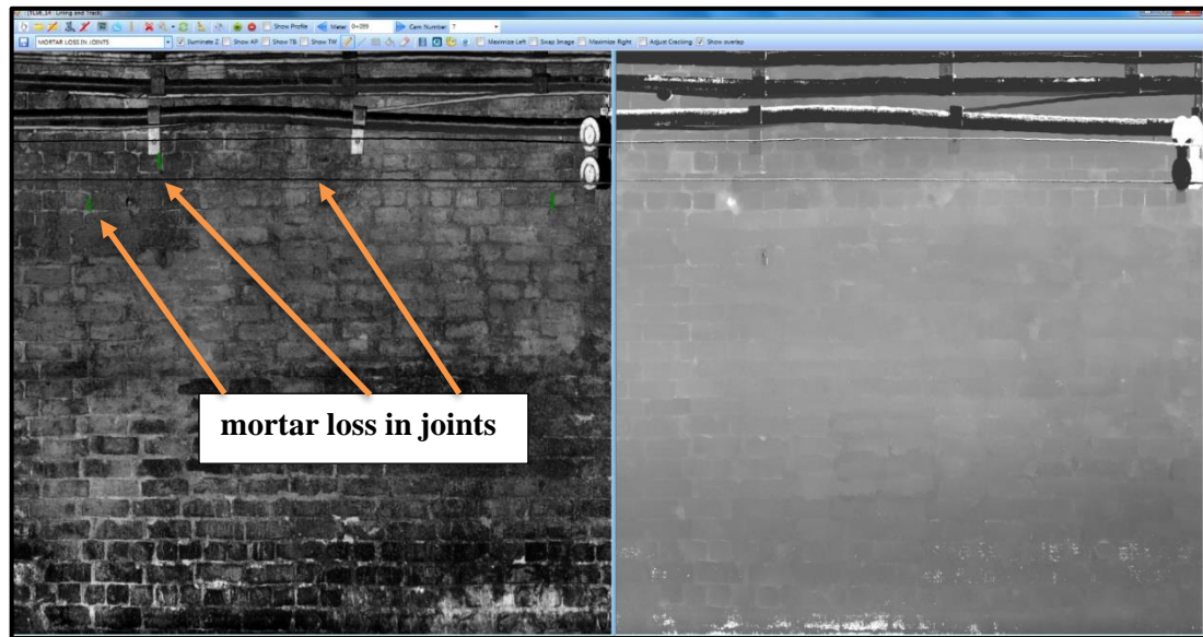
Figure 3-108 TL56 mortar loss in joints at chainage 100 2014 laser inspection
