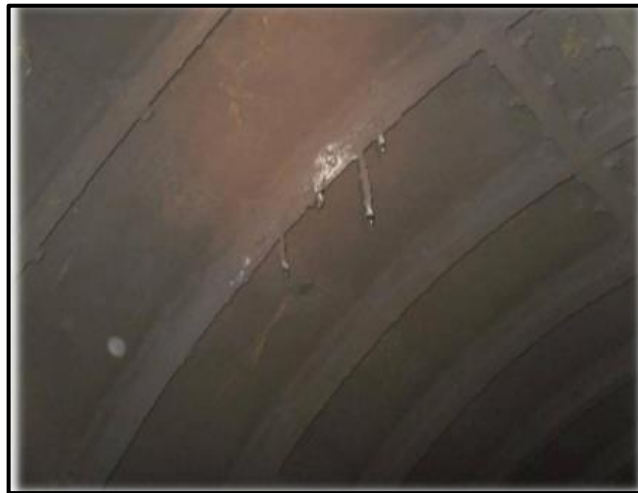
Figure 2-2 Water Ingress; harmless drip (A1)
