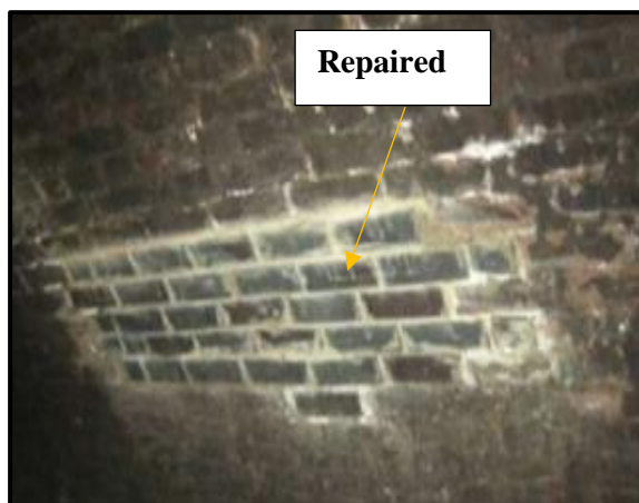
Figure 3-46 Visual Inspection Repaired area - TL56 (LUL, 2011)
