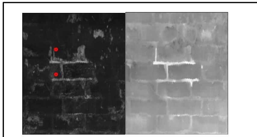
Figure 3-96 Mortar loss in joints, (enlarged)
