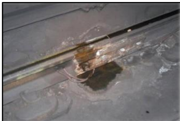
Figure 2-3 Water ingress; Rail Corrosion, Signalling fault (A4)
