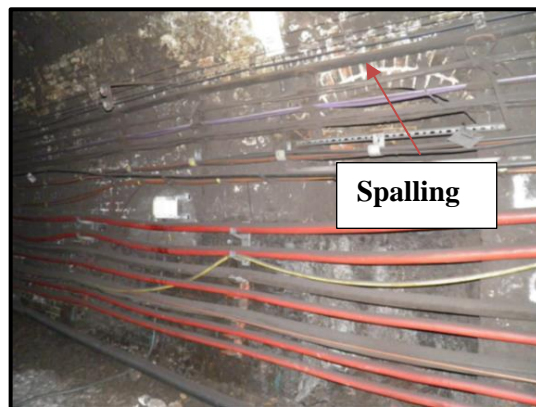
Figure 3-88 Spalling North abutment at chainage 513m from West Visual Inspection-2013
