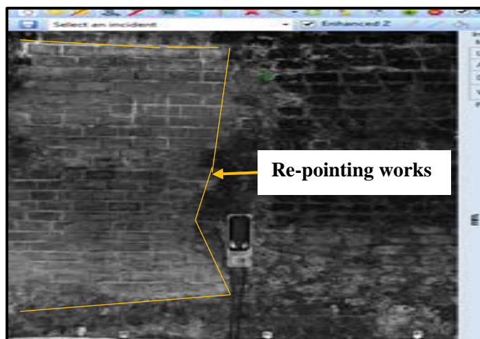
Figure 3-47 Laser Inspection Re-pointing work - TL56
