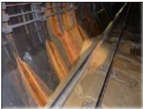
Figure 2-6 Soil ingress (C4)
