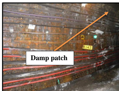
Figure 3-101 TL53 active water seepage at north abutment chainage between 95m and 100m West
