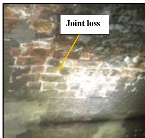
Figure 3-8 Joint loss (TL60, 2012)
