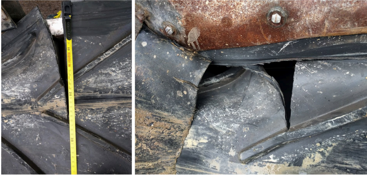
Figure 11.8: Depiction of the maximum severity of belt damage seeded to System 1 (l) and an example of loose belt material catching on hopper skirting (r).
