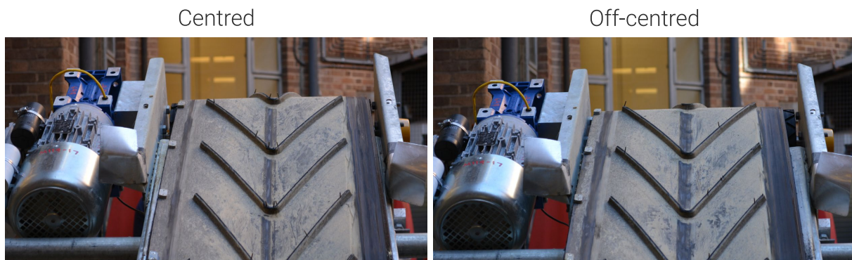
Figure 9.23: Belt tracking centred (l) and off-centred (r) at the head end of the System during CCT.F test scenarios.
