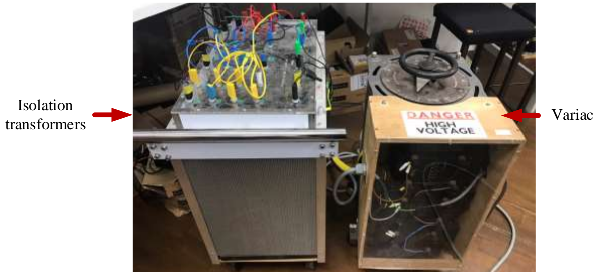
Figure 5.24 Grid-side isolation transformer as well as the variac
