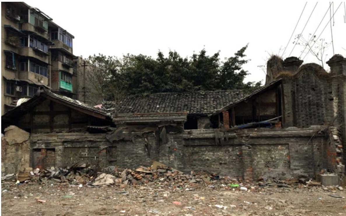
Fig. 1.5: The abandoned mansion built in 1929. Source: http://sc.news.cn/topic/lsiz2.htm
