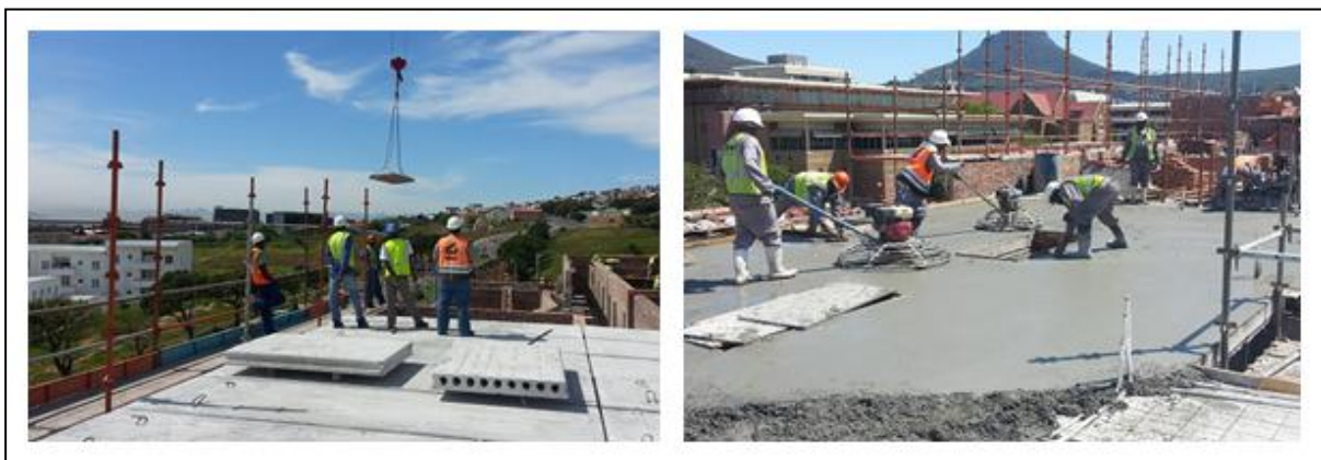
Figure 2.2: Placement of floor slabs and finishing of structural topping
