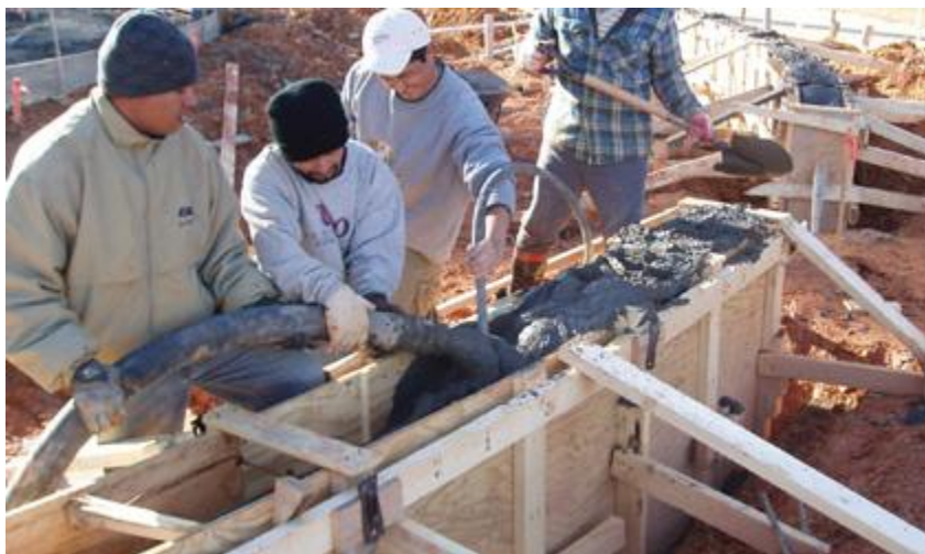
Figure 2.1: In-situ concrete construction (Concrete wall forms. 2015)
